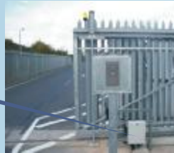
Enclosure IP-55 with toughened glass door for Motorized gate control
